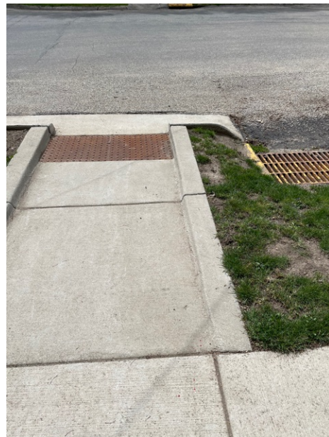
ADA compliant curb ramp on Adams St
